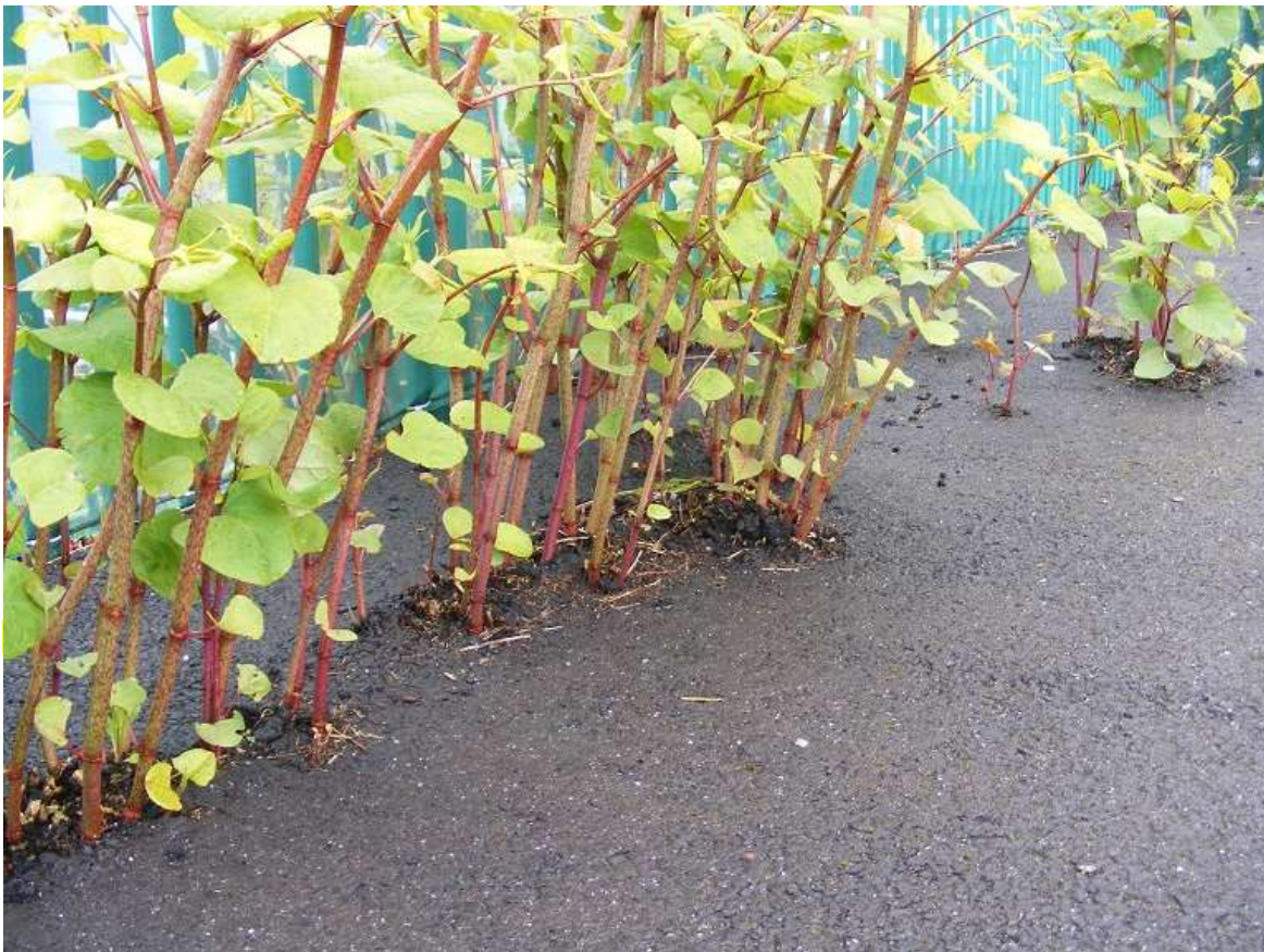
Photograph A.1 Japanese Knotweed breaking through a bituminous surface in Cork City (Source: John O' Donovan, O' Donovan Agri-Environmental Services)
